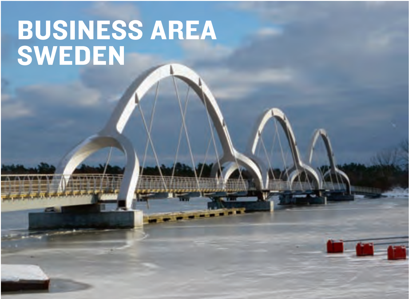
The beautiful Sölvesborgs Bridge is built from 150 tonnes of duplex steel delivered by BE Group.
